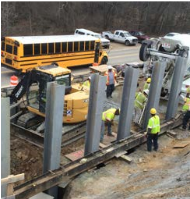
Concrete is being poured for retaining wall piles.
