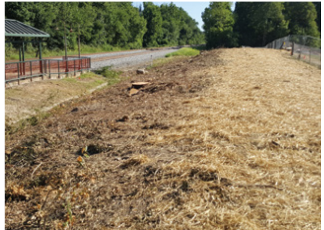
In this “after” image of the land adjacent to Lorton Station, the trees have been cleared, and the site is ready for the upcoming fiber optic relocation necessary for the extension of the existing platform.
