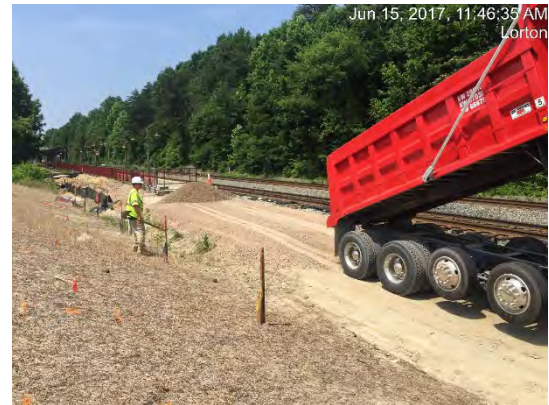
Clean fill is laid as the subgrade for the platform extension at Lorton.
