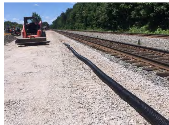
A trench for drainage is installed for the platform extension at Lorton.
