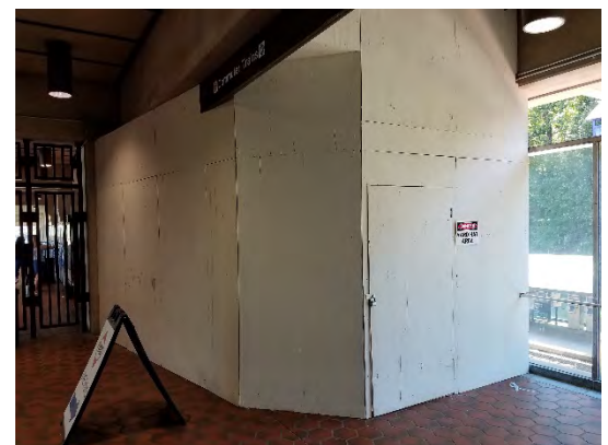
Safety Enclosure for Franconia-Springfield West Elevator Modernization
