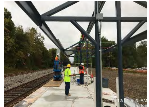
Workers erect canopy steelover the platform extension at Lorton Station.
