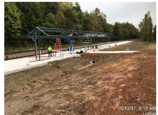
Final earthwork grading and seeding around a new entryway created at Lorton Station as part of the platform extension project
