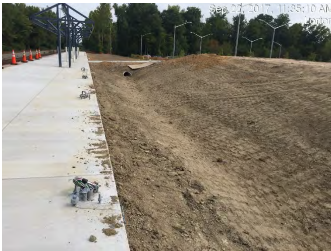
Initial grading of the drainage swale for the new platform extension at Lorton.
