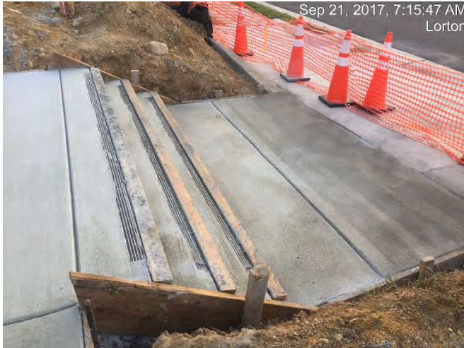
Steps are formed for the new platform entrance being added at Lorton.
