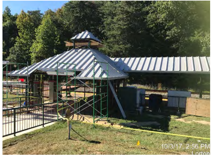
The Lorton Station Platform Extension project is also about improving the state of good repair of the existing station. The completed reroofing of the 25-year old shelter.
