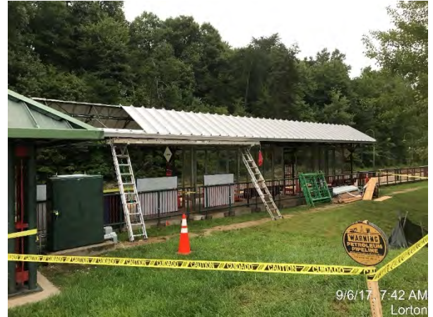
The sheet-metal roofing is replaced on the existing platform canopy at Lorton Station.
