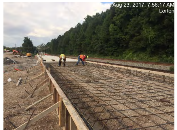
Steel reinforcing bars are laid in the forms for the new Lorton Station platform extension prior to the pouring of concrete.
