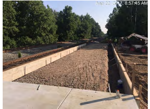
Forms are set prior to the pouring of concrete for the new platform extension at Lorton Station.
