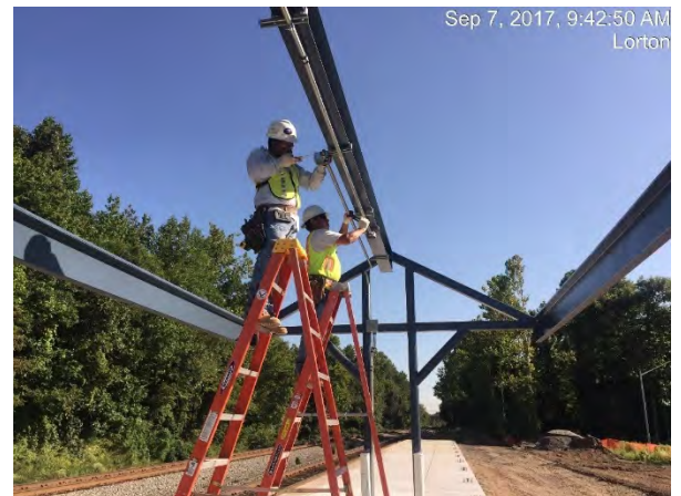
Power conduits are run through the steelwork for the new canopy on the Lorton Station platform extension.
