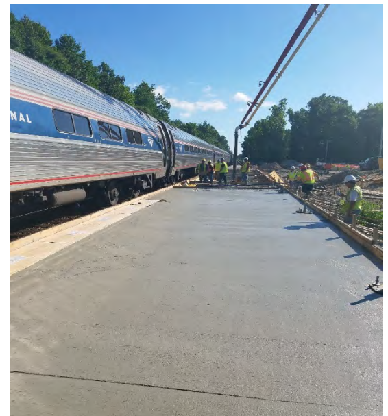
Concrete placement for the new platform extension at Lorton Station.
