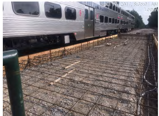
Formwork and reinforcing steel wire mesh in place for concrete placement at Lorton Station.
