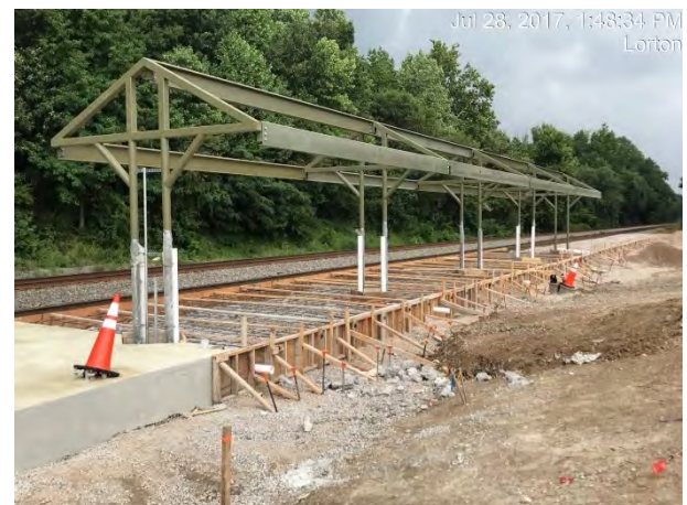
Steel erection for the new canopy as part of the Lorton Station platform extension.
