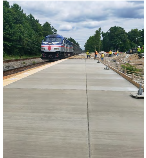
Finishing work on the new platform extension at Lorton Station.
