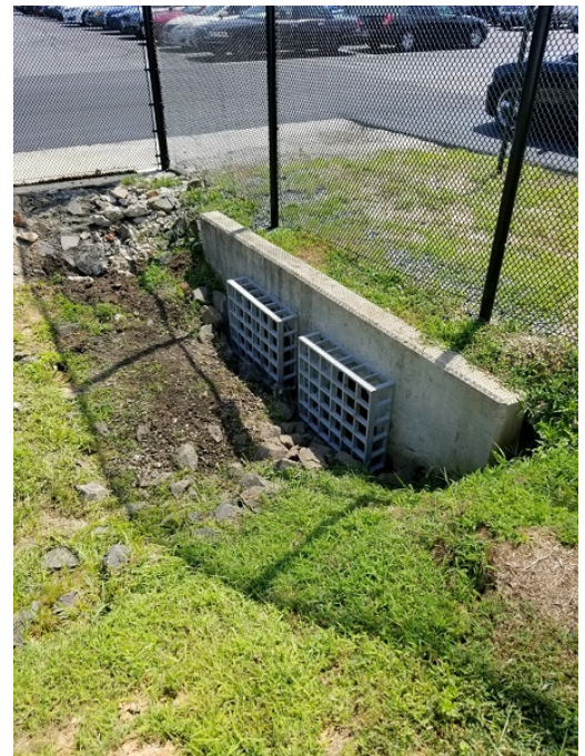
Inlet Pipe Grates at Broad Run Maintenance and Storage Facility
