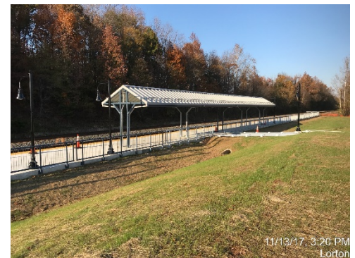
New canopy and painted railings on the platform extension at Lorton.
