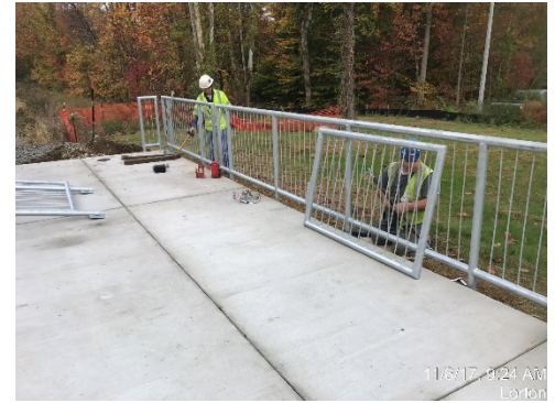
Installation of new railings the extended platform at Lorton.
