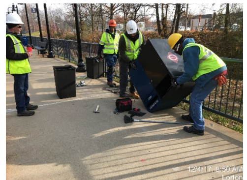
Trash and recycling can installation on the extended platform at Lorton.
