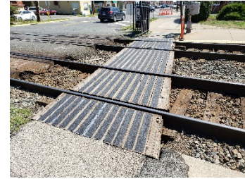
After Installation of anti-slip tape on Quantico Station pedestrian crossing
