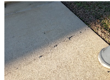
Minor cracks to be repaired on Woodbridge Station west platform
