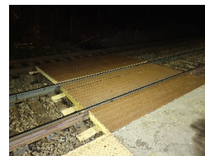
Replacement of timber crossing
