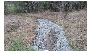
Placement of drainage stone
