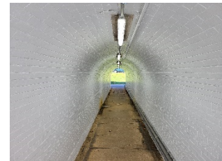
New LED light fixtures at Alexandria station tunnel
