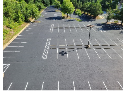
Sealcoating and restriping at Woodbridge
