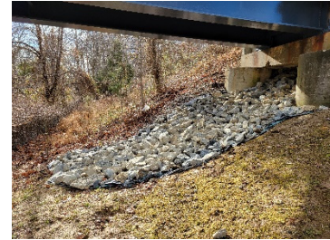
Slope protection at Rippon station
