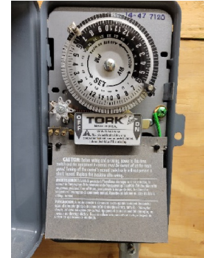
Spotsylvania station parking lot lighting time clock
