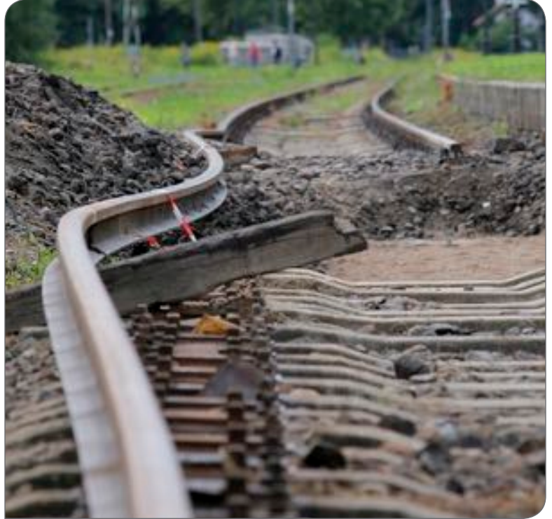
▲ Sun rail kinks are caused by a combination of heavy rail traffic and extreme heat. Photo is for reference only and is not from VRE's Host Railroads.
