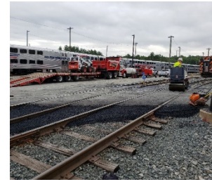
Grade-crossing paving at Crossroads as part of the LOU.
