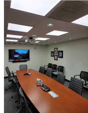
Installation of LED lighting at Alexandria headquarters
