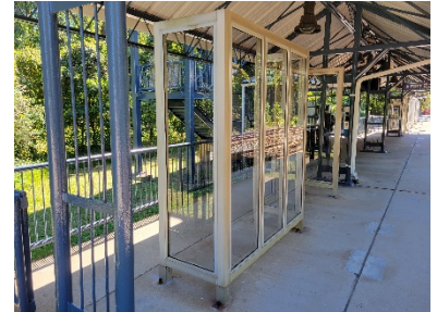
New windscreen plexiglass panels at Rippon.
