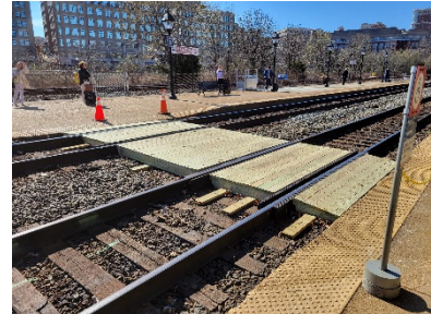
New timber pedestrian crossing at Alexandria
