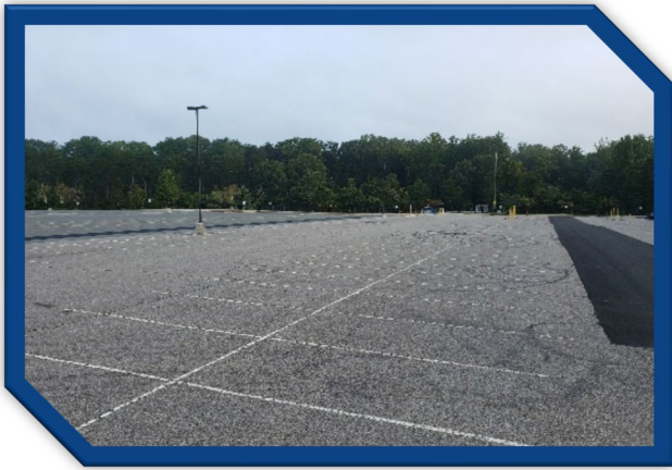
Leeland Road Station Pavement Repairs (Before)
