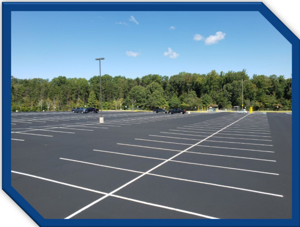
Leeland Road Station Pavement Repairs (After)
