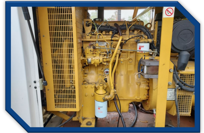
Emergency Generator Overhaul
