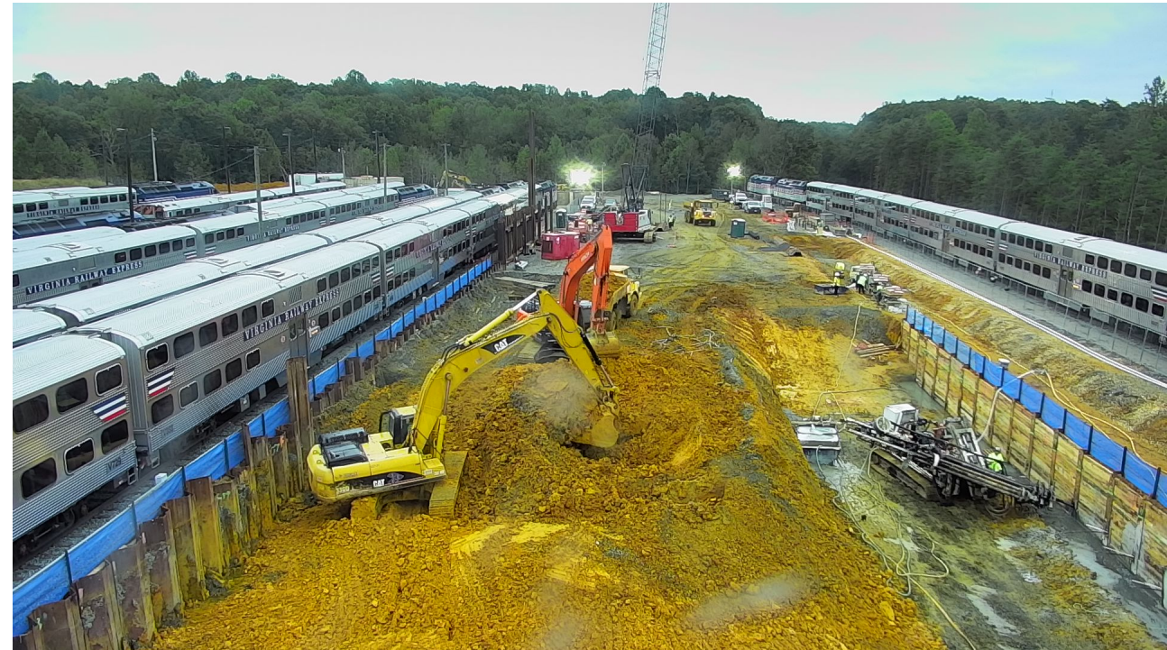
Lifecycle Overhaul and Upgrade Facility construction
